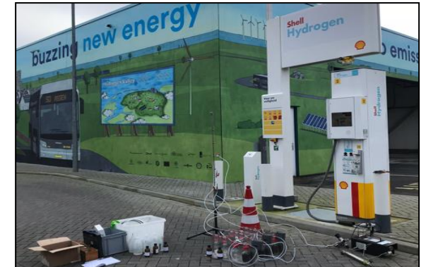
Commissioning hydrogen fuelling stations
